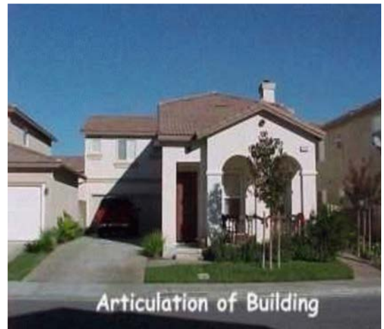
Entry Features, porch and setback garage
